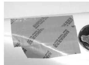
Step 2 Using a variable speed drill on the lowest speed, drill a 1/8" Pilot hole through both porcelain and metal casing of sink at the center of the desired location. (If drill bit gets hot, it may cause the porcelain to crack or chip).
