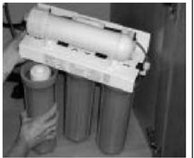
Step 5 The sediment filter has a cloth-like appearance. It must be in the FIRST housing on the left (where the water inlet connects).
