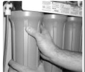
Step 4 Clean all filter housings with a mild soap solution and rinse with water. Check O-rings and lubricate with water soluble lubricant. Water based lubricants can be used, but petroleum based lubricants (such as Vaseline) must not be used.
